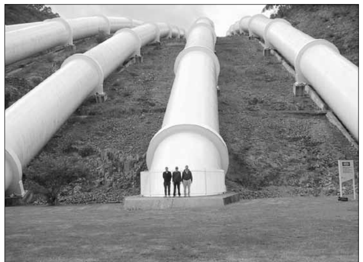
The six pipes of Tumut 3 are each 487 metres long, 5.6m in diameter, and collectively contain 10,260 tonnes of steel. Photo: Gabrielle Peut
