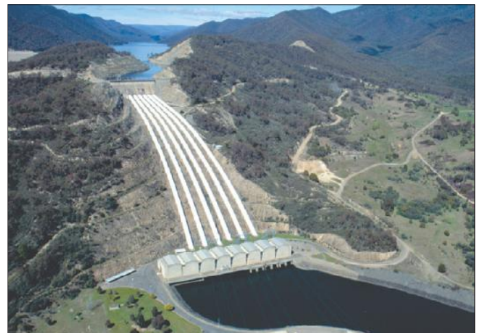
Projects like the Snowy Mountains Scheme, were conceived by visionary nation builders, which Australia sorely needs today. Photo: Snowy Mountains Hydro-Electric Authority
