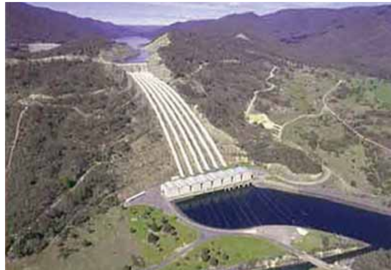
Huge pipes carrying water to turbines in the Snowy Mountains Hydroelectric Scheme, the one great Post-War Reconstruction project not squashed by the City of London.
